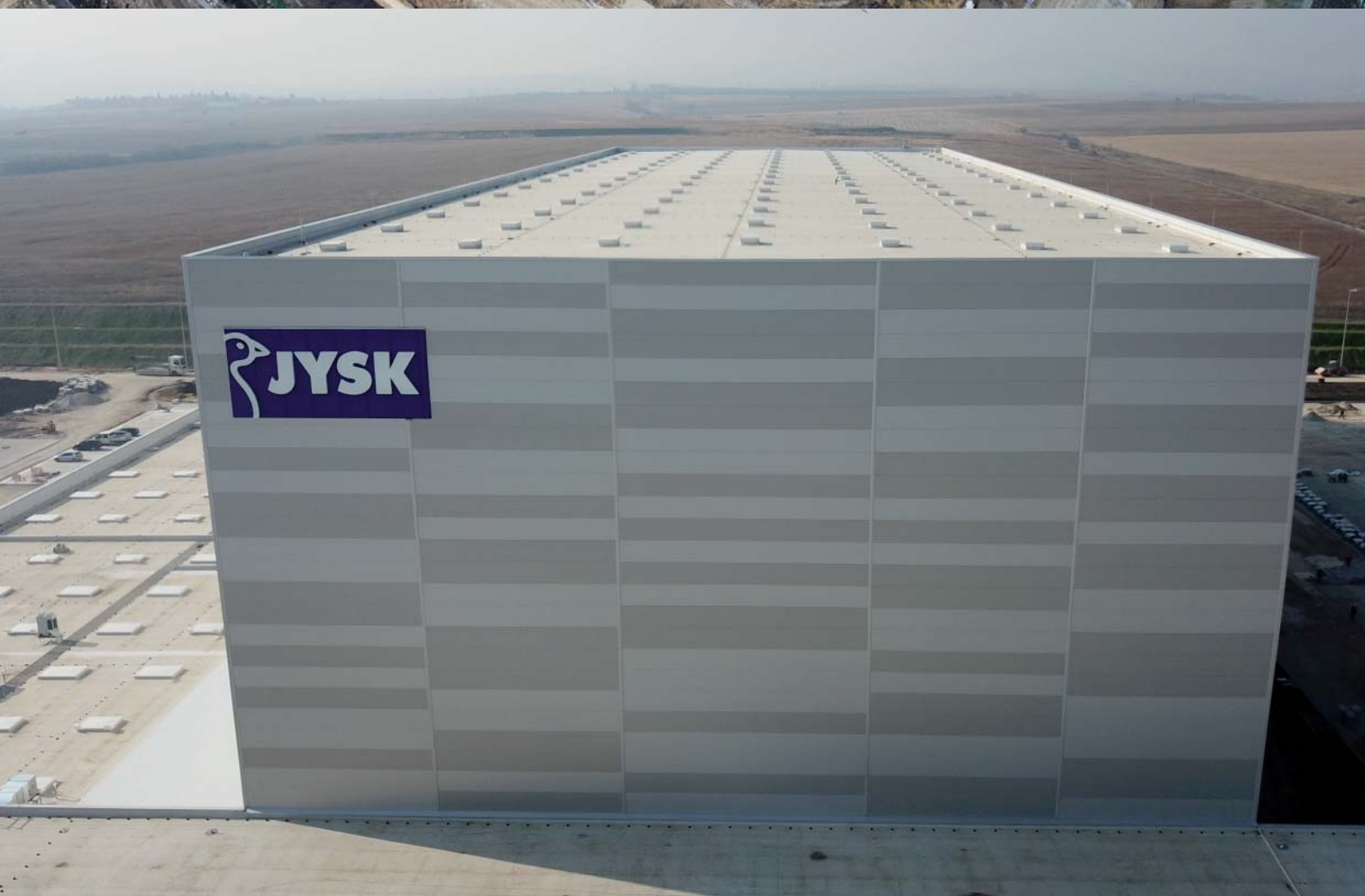
The SHEV systems generate an effective opening area of 97 m 2 for each of the two high-bay storages.
