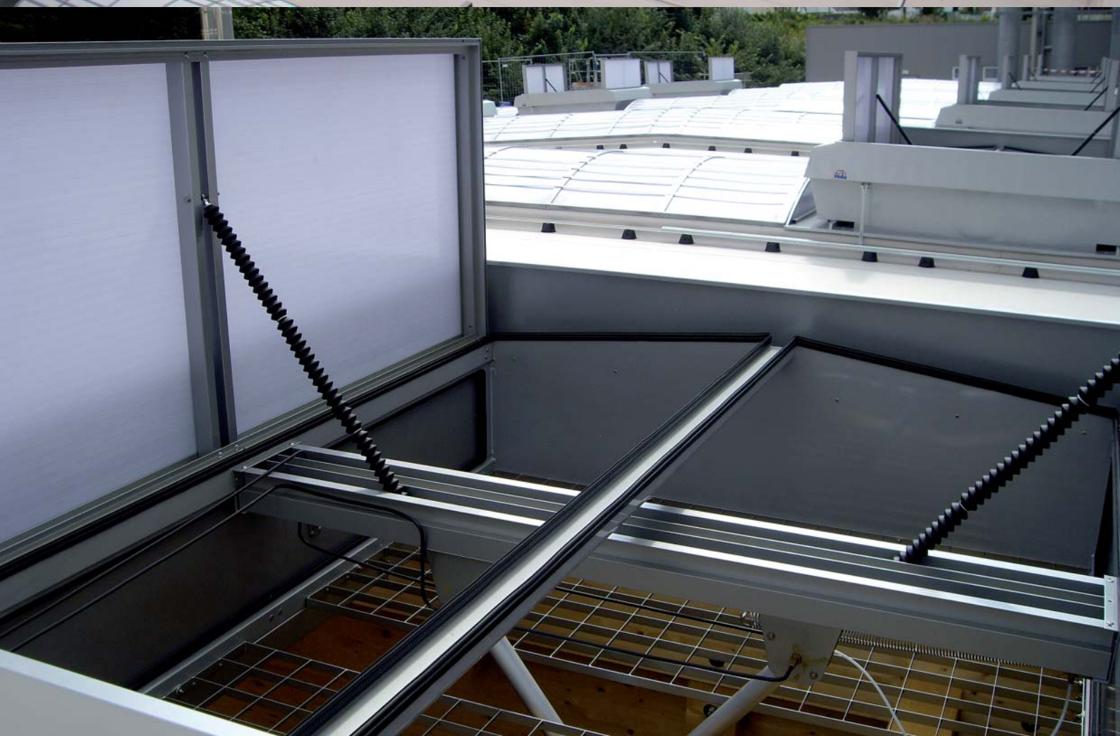
Special cylinder with bellows and hard chrome-plated piston rod. Feeds within the system are made of plastic.
