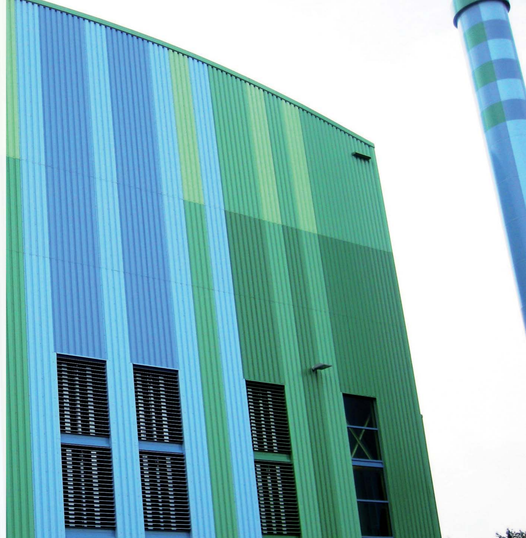
Large illustration: AIRJET air inlet unit with splitter attenuators mounted behind it.
