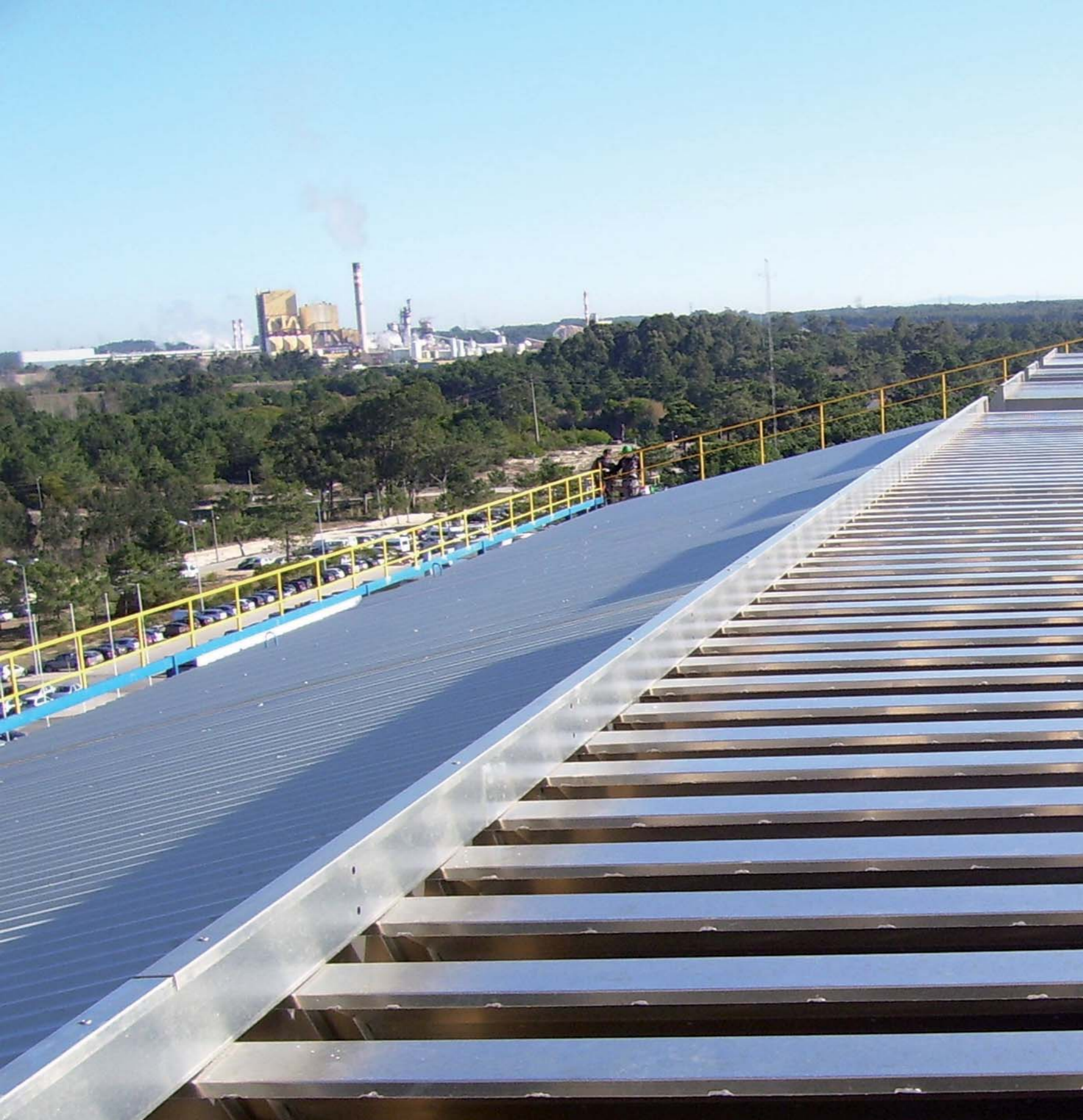
Large illustration: AIRSTAR labyrinth ventilator spread along the whole ridge of a factory building.
