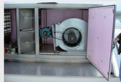
Ventilator module with a radial fan
