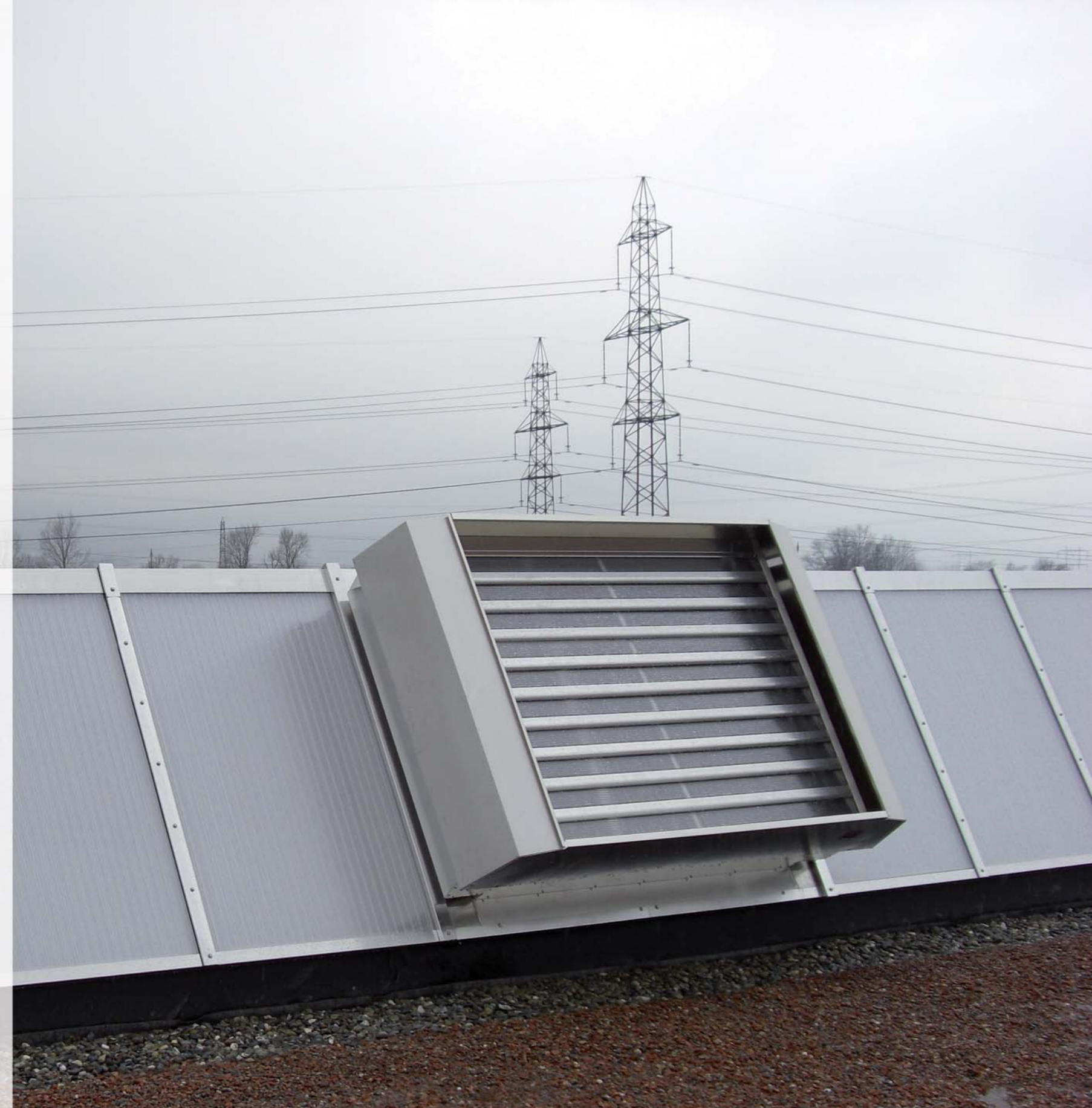
Large illustration: MULTIJET with polycarbonate louvre blades mounted in a DELTALIGHT.
