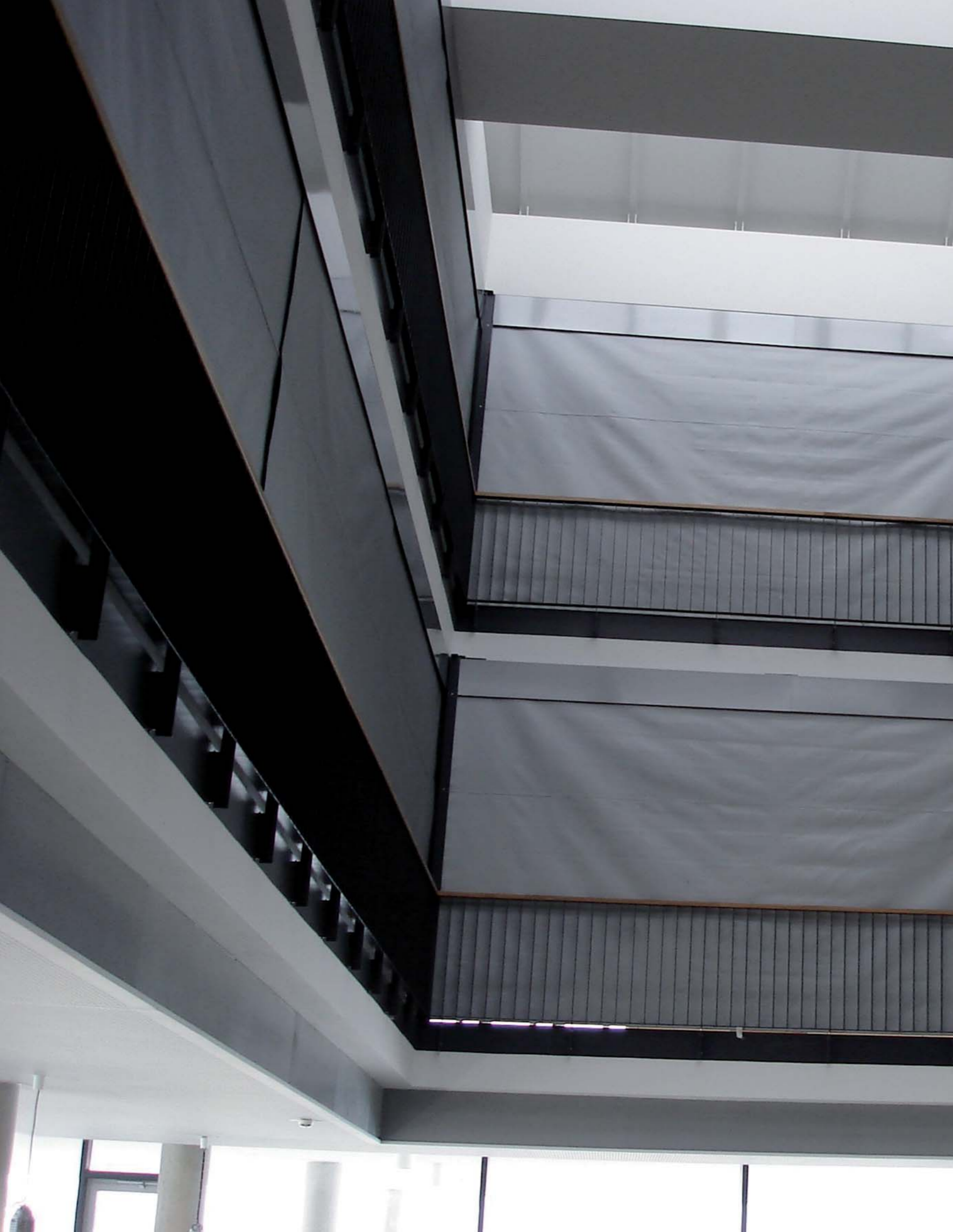
Picture: Rolled smoke curtains for channelling the smoke in a stairwell
