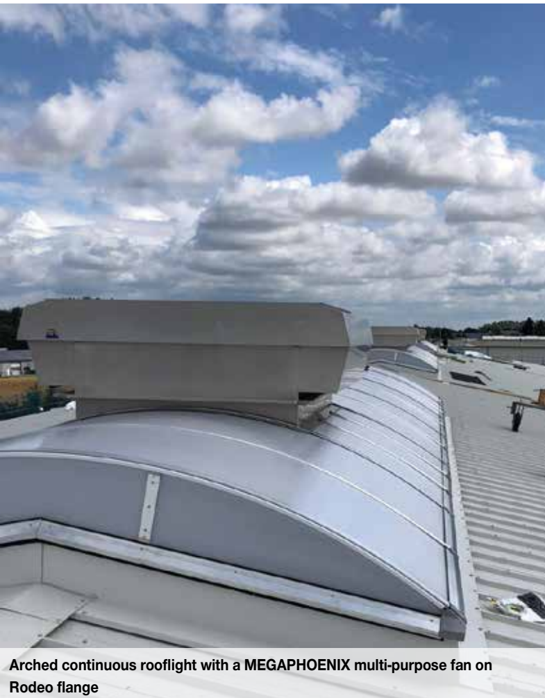
Continuous rooflight with MEGAPHOENIX multi-purpose fan
