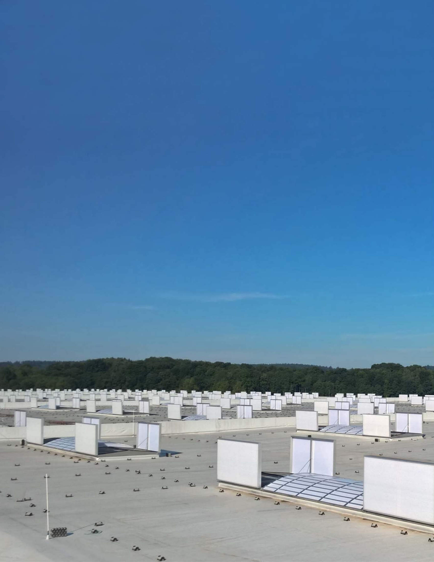
Illustration: EUROLIGHT roof lights with a total of 180 PHOENIX NSHE installed on top of the roof of a logistics centre.
